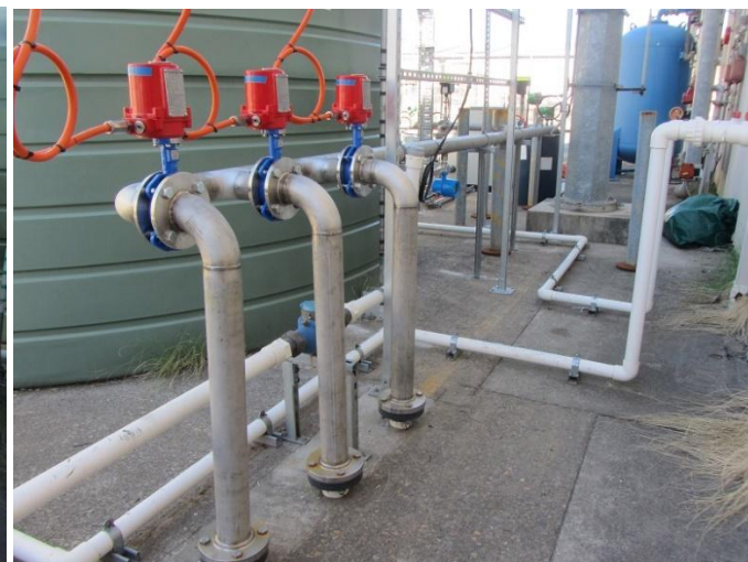
Photo 2: Valves directing air to the three sections of the aquifer.
