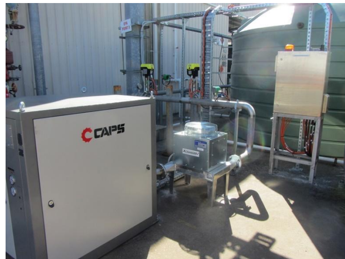
Photo 1: Blower, cooler, control cabinet and piping.
